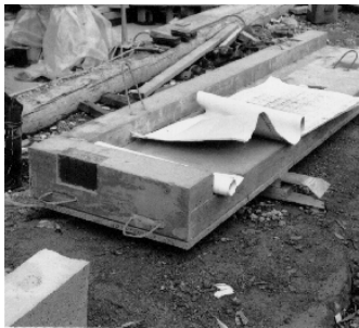
Figure 13. Franklin Square Pre-cast element with granite facing (Hartman-Cox, Architects)
